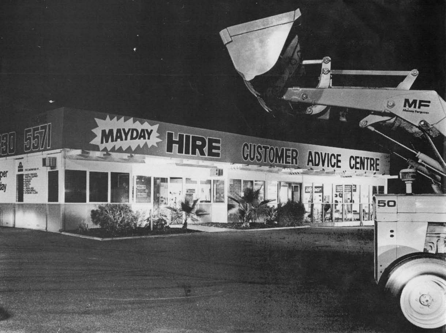
Mayday's new Customer Advice Centre, Leach Highway, Melville, W.A. is reported to be the largest of its kind in Western Australia, with a display area which totals 1½ acres.
